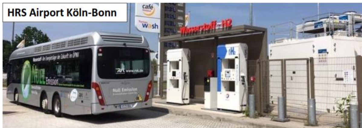
Figure 17. Upgraded HRS with additional dispenser at Köln-Bonn Airport (source: H2M)
