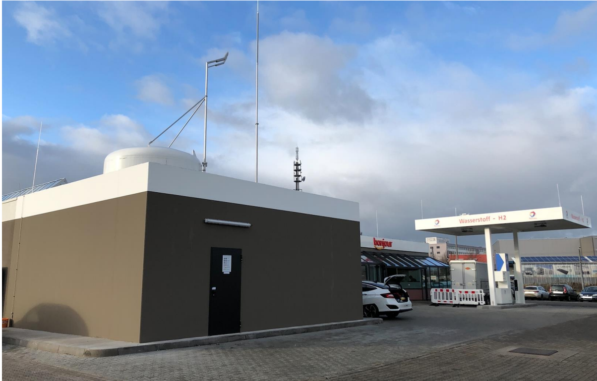
Figure 14. Erfurt HRS enclosure (including LH2 storage) and dispenser pictured during commissioning (source: H2M)
