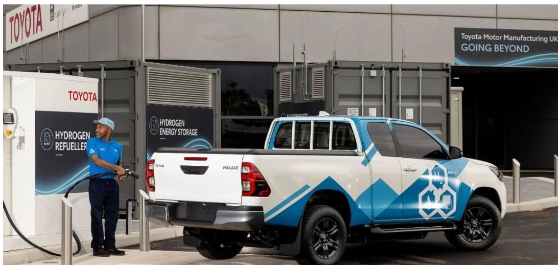
Figure 16: Fuel Cell Systems Hydrogen Refueller at Toyota Burnaston
